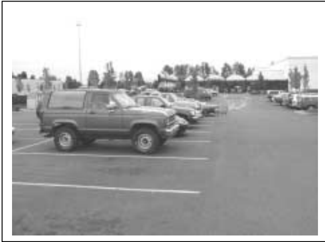
Figure 4. In this parking lot with 19-foot deep parking spaces and 24-foot wide aisles, most cars do not fill the parking spaces, as shown by the alignment of cars parked on the left side of the picture. Unfilled parking spaces add to the effective width of the aisle for maneuvering, though the painted striping defines the driving area.
