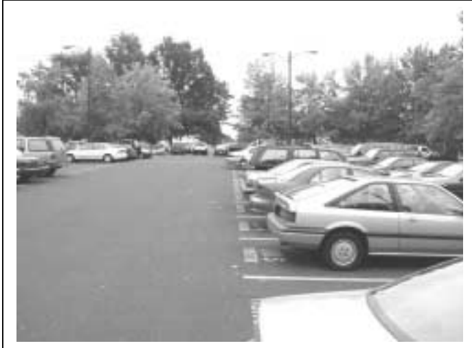
Figure 5. This parking lot has parking spaces 16 feet long by 8 ½ feet wide, and 24-foot-wide aisles. Only one car in this row extends into the aisle (the white car in the background). These spaces do not overhang landscaping, so this picture shows how cars will fit into a 16-foot deep parking space.
