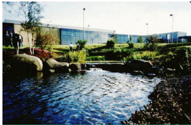
**Stormwater wet ponds are characterized by a permanent pool of water.**
