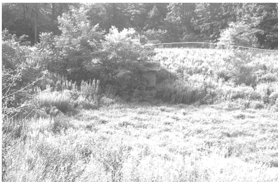
Stormwater management pond lacking effective maintenance
