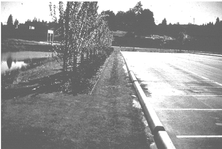
Curb cuts allowing water to pass across the vegetative filter strip prior to exiting the site thus disconnecting the impervious areas
