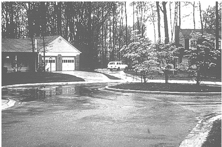
Typical Cul-de-Sac where the center area is made pervious which reduces overall site Imperviousness
