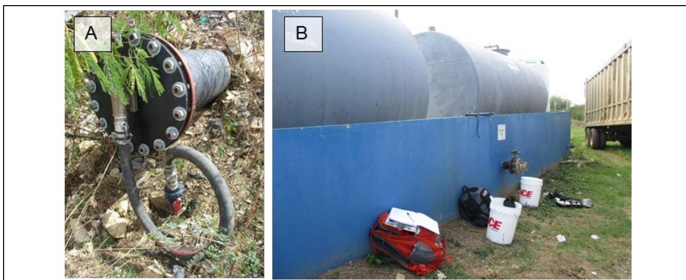
Figure 3.3. 5,000-gallon leachate tanks: intake (A); outlet (B).
