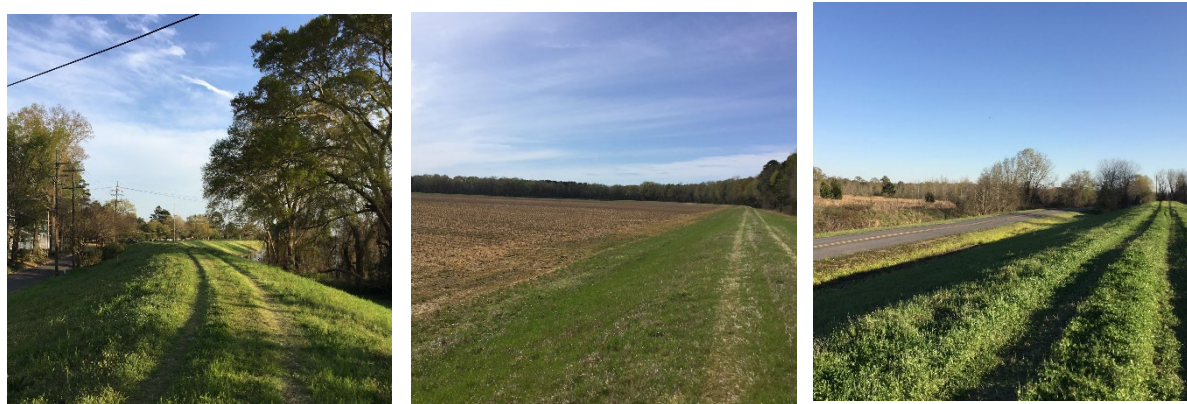
Figure 1.2 Ouachita River Levee. Photo credit: Ouachita Parish Police Jury
