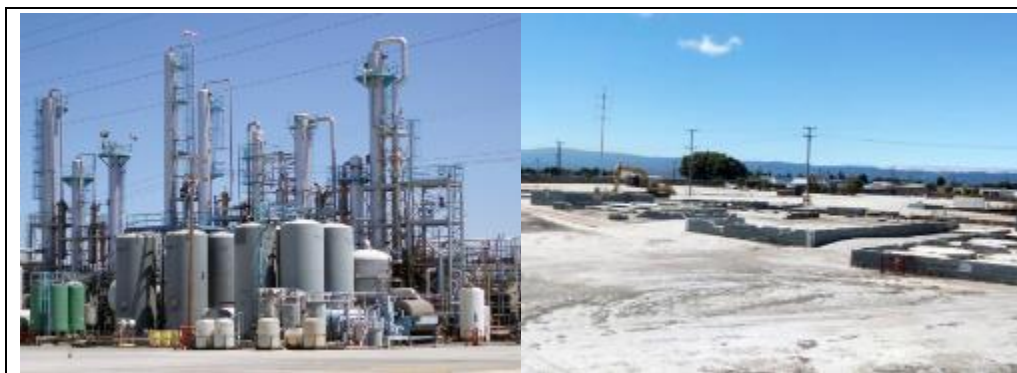
The Bay Road Holdings site in 2008 (left) and after demolition in 2017 (right). (US EPA, 2018c). Remediation of subsurface solvent contamination is ongoing via a groundwater recirculation system with horizontal injection of a sugar-based substrate.
