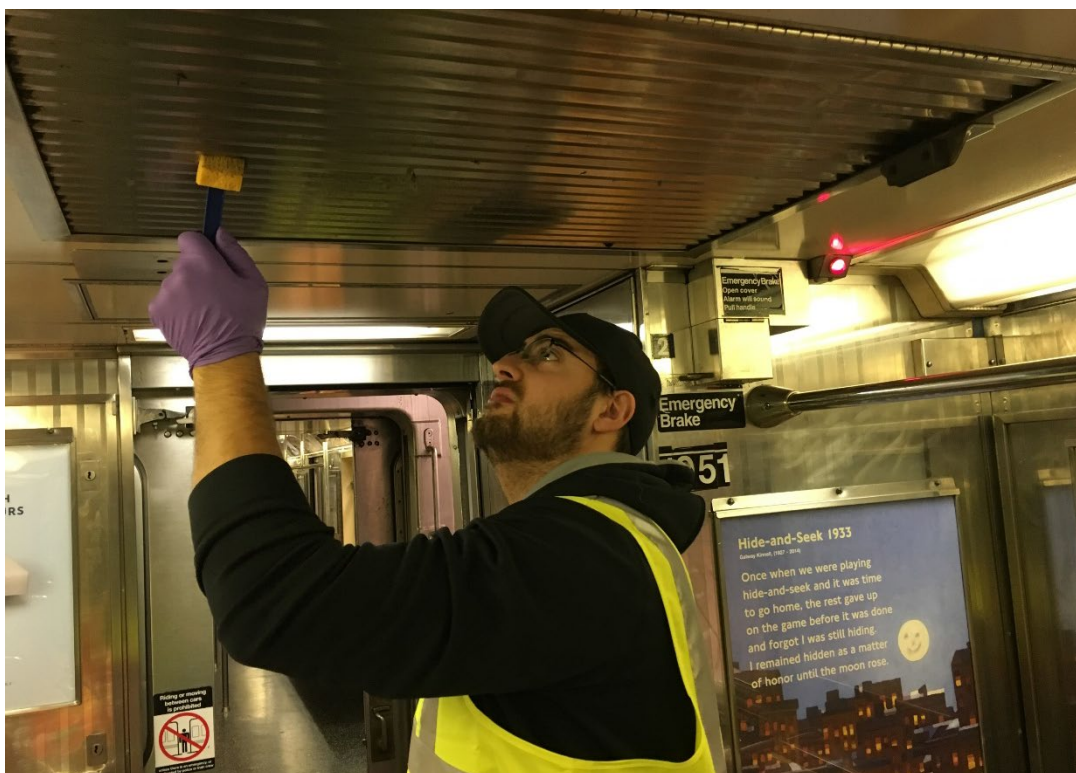
Figure A-19. Subway Car Filter Grille Located on the Front and Back HVAC Returns of Car 1951 – Sampled with Sponge-Sticks
