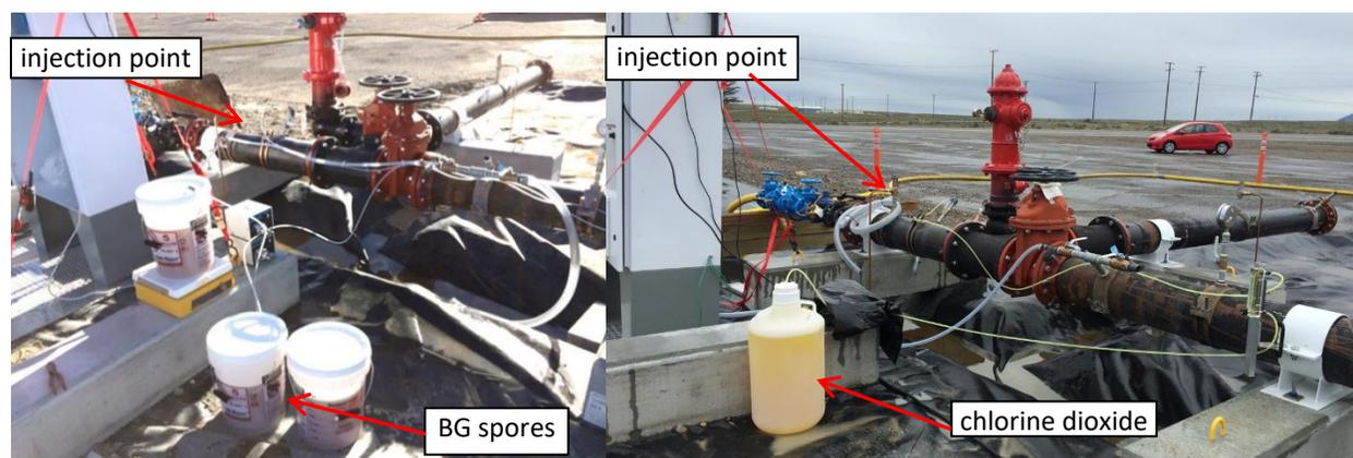
**Figure 2: Injection of *Bacillus* (BG) spores (left) and chlorine dioxide (right) into the pipe.**
