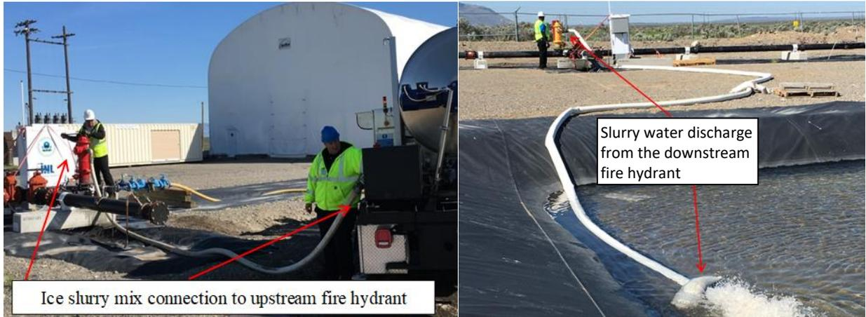
**Figure 4: Ice pigging taking place by pumping an ice slurry down the Water Security Test Bed pipe.**
