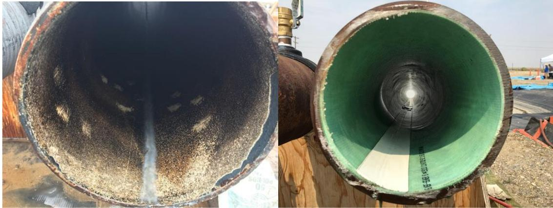
**Figure 7: Pipes lined with Oceanit DragX (left) and CIPP (right).**
