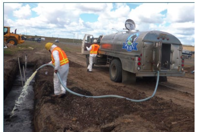
Cheese whey being applied during the construction of the sustainable bioreactor demonstration project. Fairchild AFB worked cooperatively with a local creamery to enable the reuse of cheese whey, a byproduct from creamery processes. The cheese whey served as a necessary carbon source within the construction of the solar-operated bioreactor and promotes the breakdown of contaminants in groundwater and using natural processes. (Figure source: Secretary of Defense, 2012).
