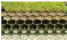
Figure 4-14: Reinforced grass paving allows water to pass through the grass' root zone and into the underlying soil while still maintaining a hard surface for vehicular travel.
