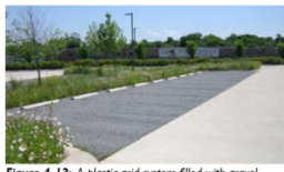
Figure 4-13: A plastic grid system filled with gravel provides the structural strength to support a vehicle.
