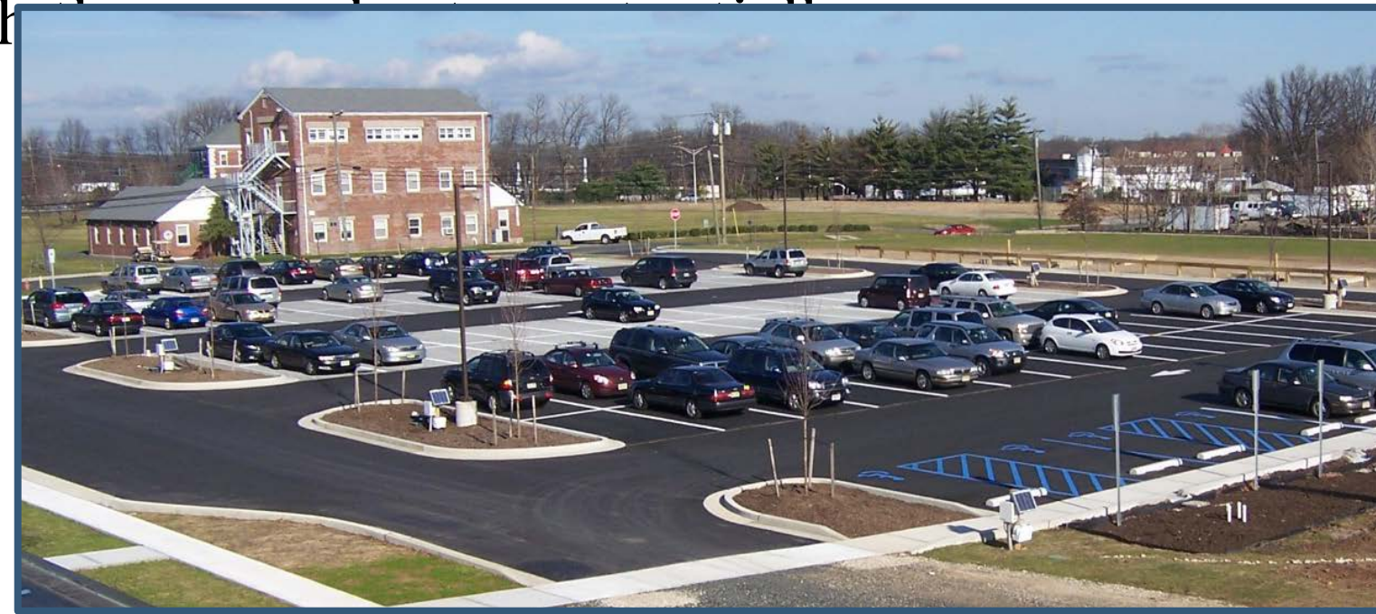
Permeable parking lot, Edison, NJ
