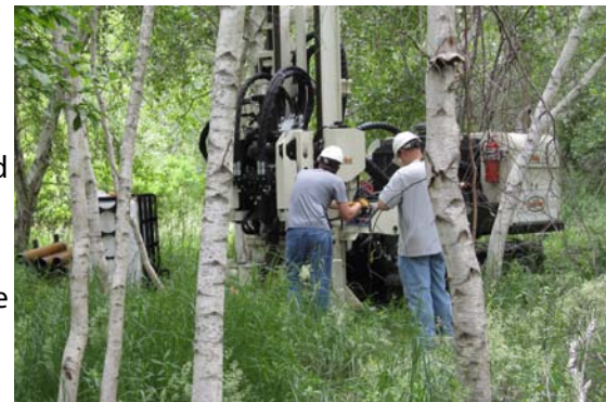
GWERD scientists installing monitoring wells.
