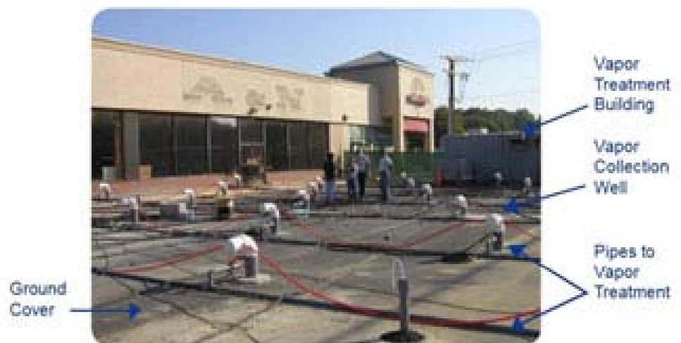
An electrical resistance heating (ERH) thermal treatment installation.
