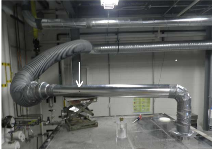
Figure 6.2-2. Test Chamber Exhaust Duct (white arrow shows sampling point location)
