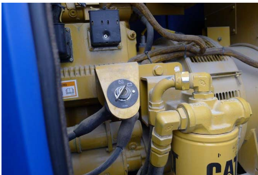
Figure 14. Connect Battery in Preparation for Starting Generator
