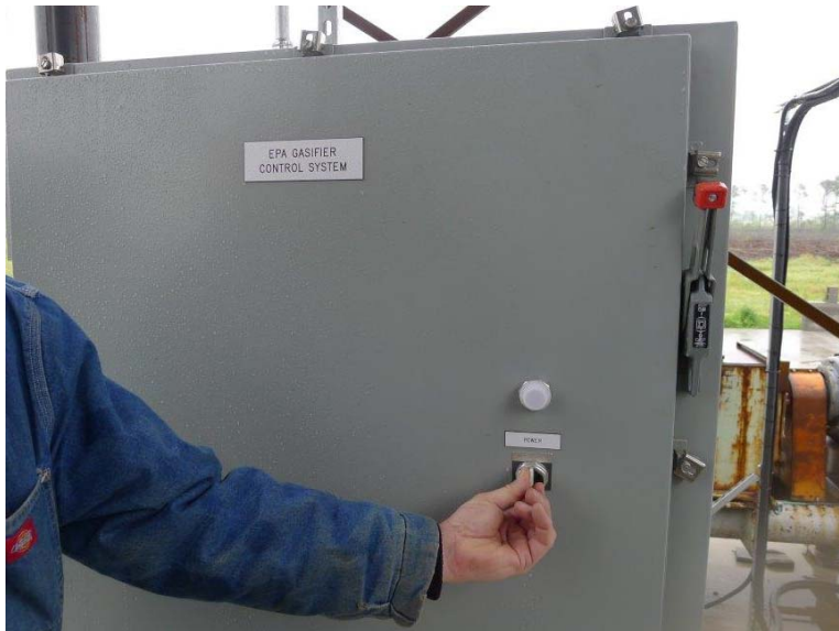
Figure 20. Power Switch on EPA Gasifier Control Panel
