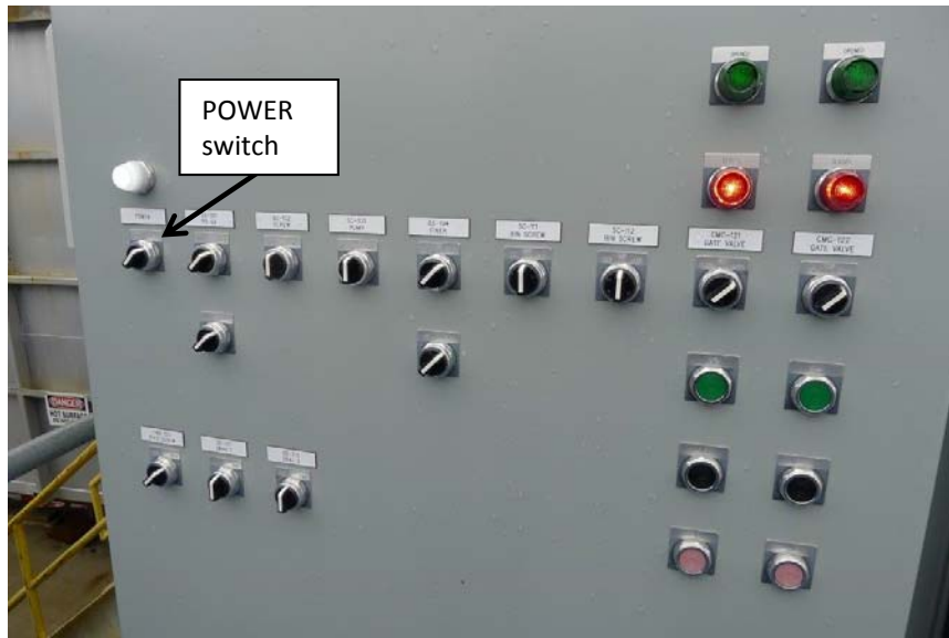
Figure 17. Power Switch on front of Power Distribution Panel
