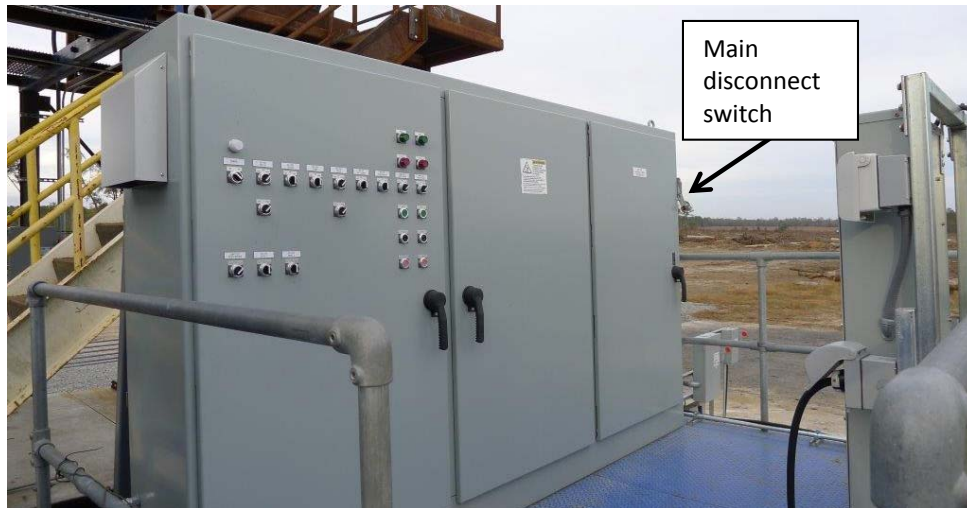
Figure 16a. Outside of Power Distribution Panel
