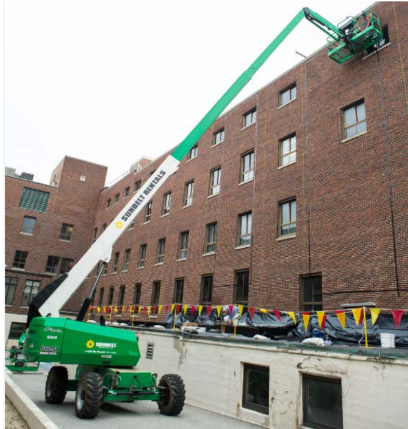
Figure 4. Twenty-meter boom lift that was used to reach the higher elevations safely during the scalability demonstrations.
