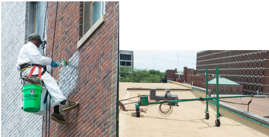
Figure 5. Bosun chair (left) and deployment from building roof (right).
