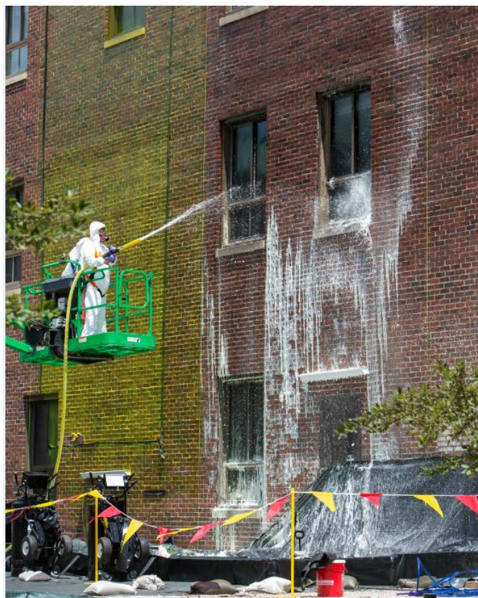
Figure 19. A water rinse was applied to remove UDF.
