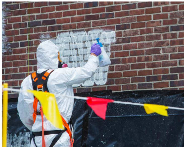
Figure 18. UDF containing the oxidizer was applied to a small area using a handheld sprayer.
