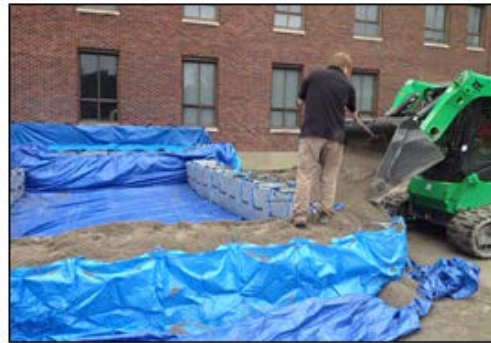
Figure 36. As seen in the images above, a ground liner was laid out, and then the HESCO® barrier units were assembled on top of the liner (top left). A skid steer loader was used to build the earthen berm for driving into the containment (top right) as well as to load sand into the assembled baskets (center). The HESCO® barrier units continued to be assembled and filled to create a containment berm (bottom two photos).
