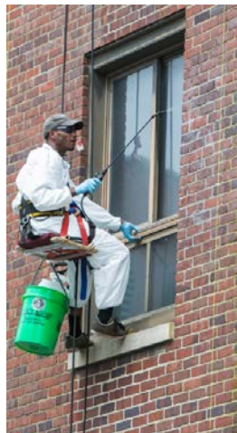
Figure 24. SuperGel was removed from the wall using a water rinse from a hand held sprayer.
