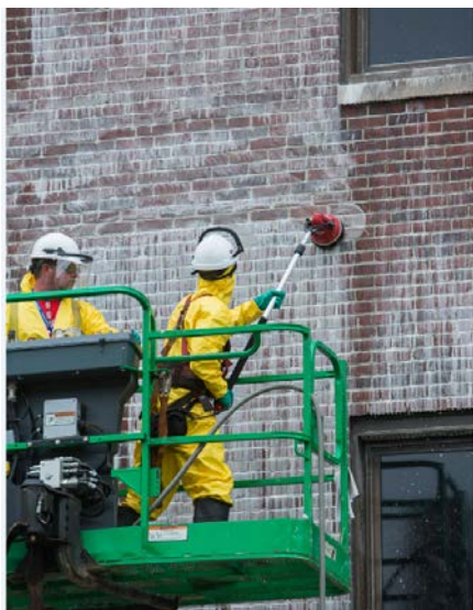
Figure 13. A battery powered rotating scrub brush was used after application of Rad-Release II Solution 1 and Solution 2.
