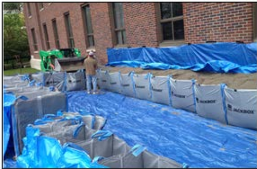
Figure 36. As seen in the images above, a ground liner was laid out, and then the HESCO® barrier units were assembled on top of the liner (top left). A skid steer loader was used to build the earthen berm for driving into the containment (top right) as well as to load sand into the assembled baskets (center). The HESCO® barrier units continued to be assembled and filled to create a containment berm (bottom two photos).
