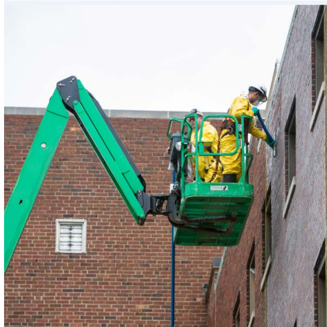
Figure 10. Attempting to vacuum SuperGel. Vacuum hose kept clogging.
