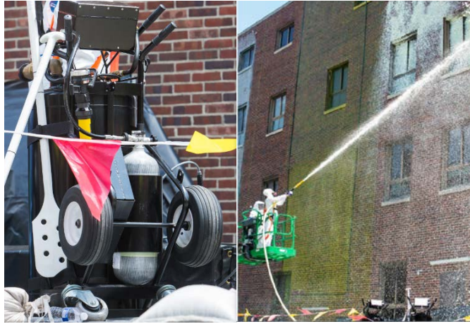
Figure 17. Air Foam Dolly System (left) used for UDF application (right).
