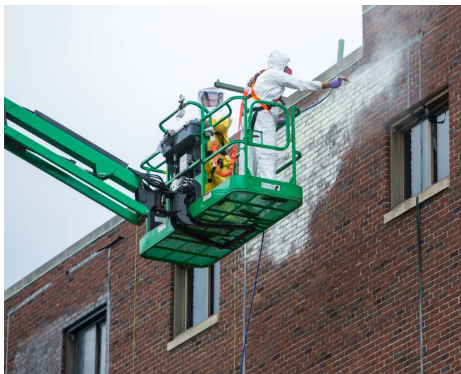
Figure 7. Stripcoat application via sprayer.
