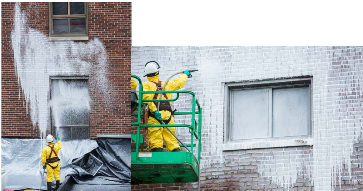
Figure 12. Application of Rad-Release II Solution 1 from the ground (left) and lift (right).
