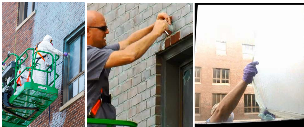
Figure 6. Application of DeconGel (left), attempted removal of cured DeconGel (which is non-hazardous) from brick and mortar (middle), successful removal from window glass (right).
