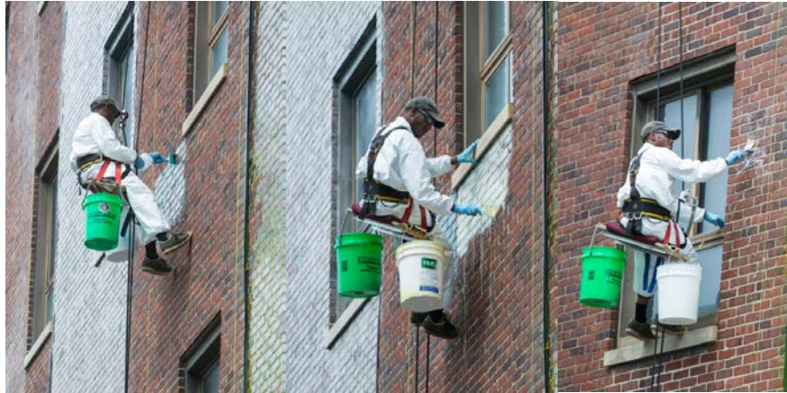
Figure 22. Bosun chair application of DeconGel (left), Stripcoat (middle) and SuperGel (right) using a paint brush.
