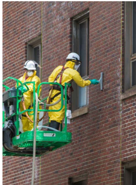
Figure 15. After water rinse was applied, the Rad-Release II was vacuumed.
