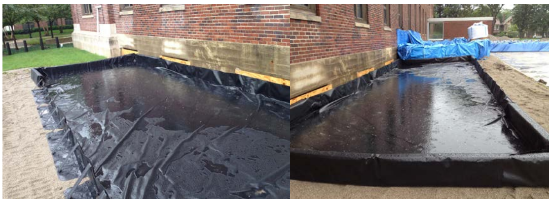
Figure 30. Building containment berms.
