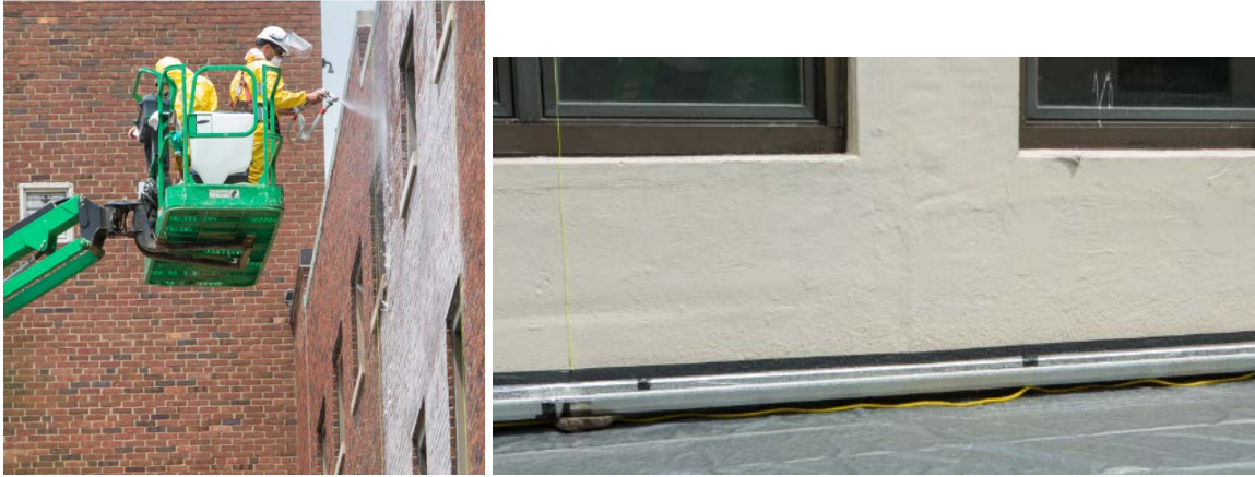
Figure 11. Applying a water rinse for SuperGel removal (left) and an aluminum gutter system at base of building for SuperGel and rinse water containment and collection using a vacuum (right).
