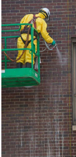
Figure 14. Water Rinse of Rad-Release II Solution 1.
