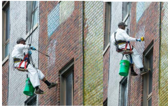
Figure 23. Bosun chair application of water simulation of Rad-Release II with a hand sprayer, followed by hand scrubbing.
