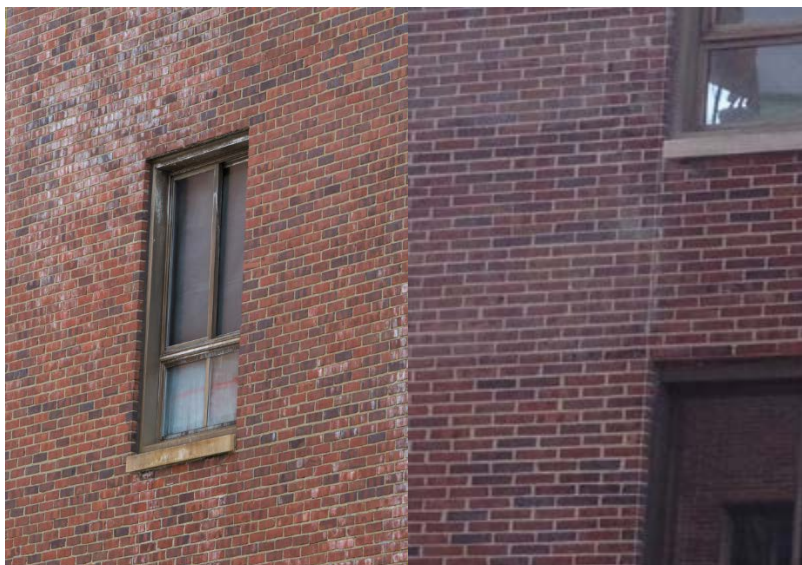
Figure 16. Brick took on a white “chalky” look after water rinse and vacuum removal steps of Rad-Release II. Image on left was taken a few days after demonstration, and image at right was taken two months after demonstration. Staining is evident as brick between windows in right image remained untreated while that to the left of the vertical line is clearly still stained (different shade of overall brick color is due to the lighting when the picture was taken).
