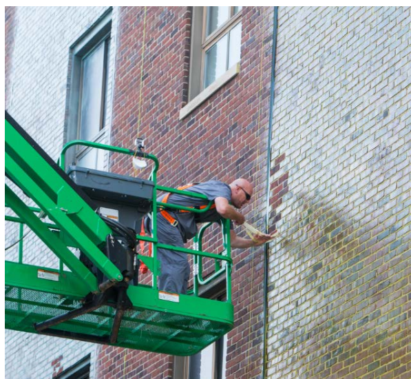
Figure 8. Removing Stripcoat by hand, peeling it off of the wall (cured material is non-hazardous).
