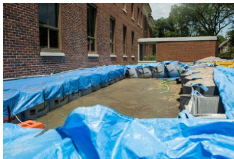
Figure 35. Images show the floor of the HESCO® berm for the building containment. Each unit was filled with sand and then covered with a tarp.
