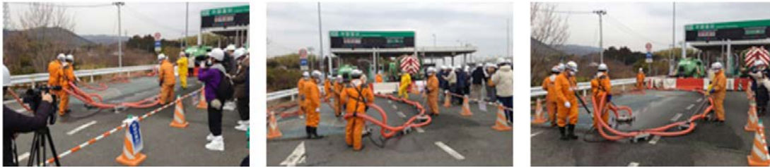
Figure 2-15. Spin-Jet Decontamination of the Jōban Expressway (recreated from MOE) 10
