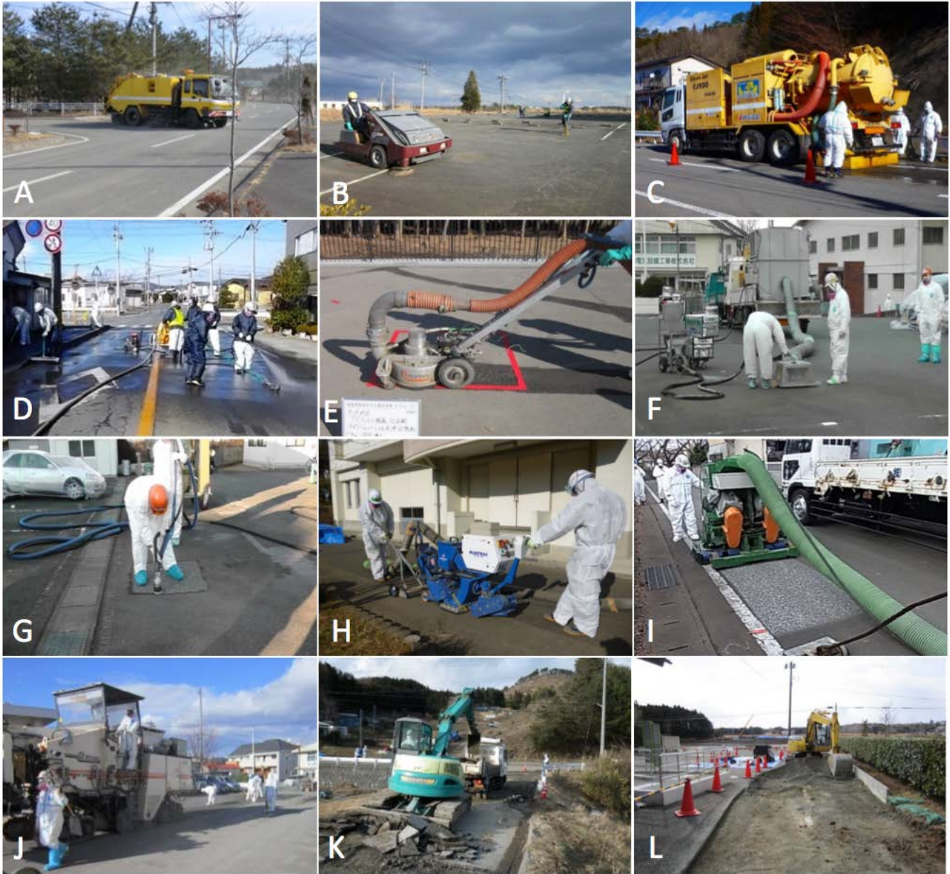
Figure 2-14. Example Road Decontamination Techniques (recreated from JAEA, 2015a)
