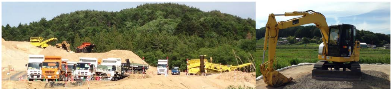
Figure 2-20. Excavation of Topsoil and Vegetation
