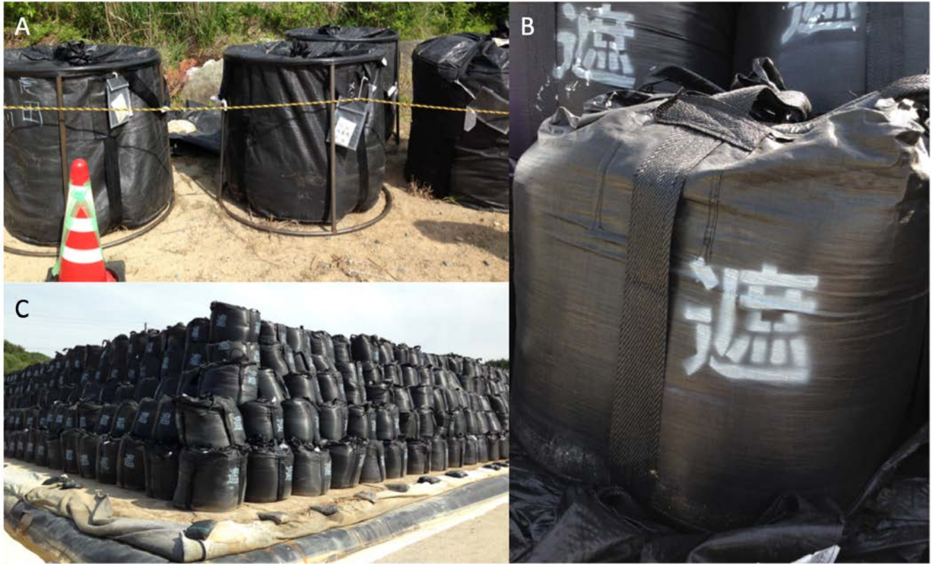
Figure 2-21. Contaminated Soil and Vegetation Waste Containment
