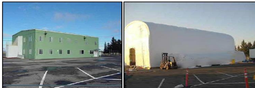
Figure 1. Two story building, without and with secondary containment (tenting), at Idaho National Laboratory.
