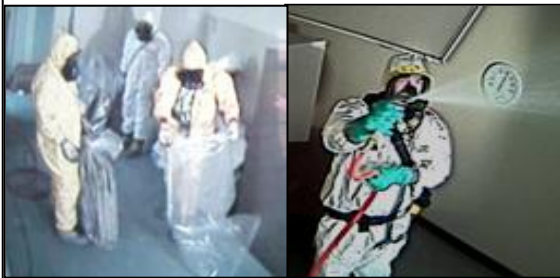
Figure 5. Bagging porous materials (R) and spraying with pH-adjusted bleach (L).
