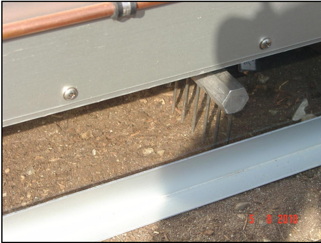
Figure 11. Uneven surface beneath tunnel wall must be relatively even to eliminate the release of air from beneath the frame.
