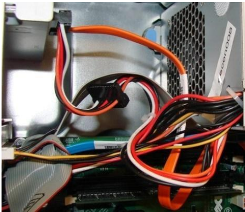
Figure 4. Unaffected Internal Wires (75 ppmv)
