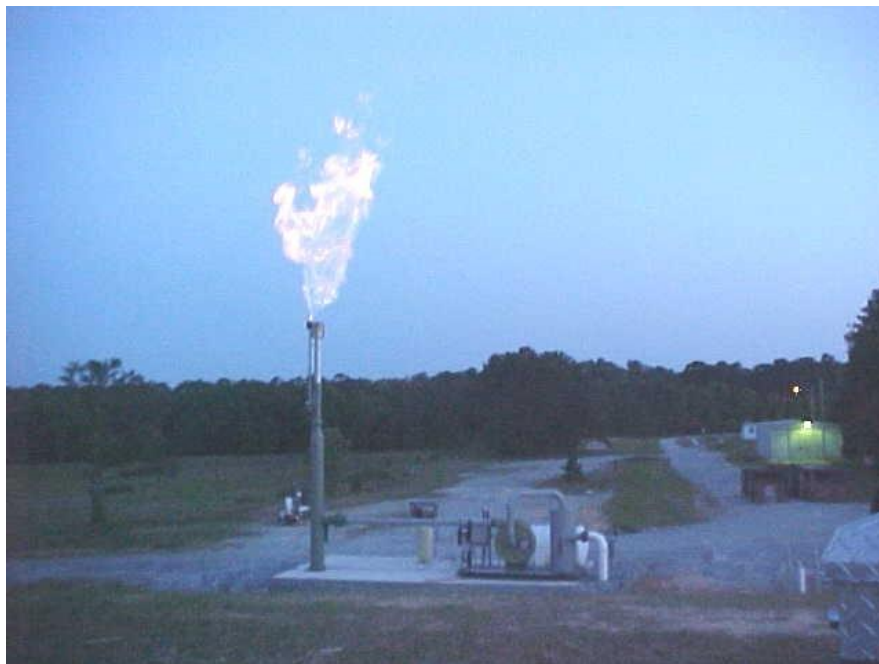
Figure 3. Collection System & Flare (subsequently fenced)
