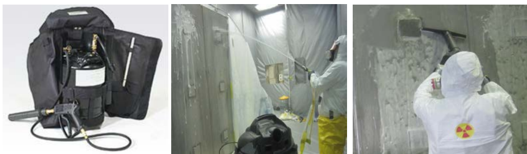
Figure 3-3. Backpack foamer, foam application, and vacuum removal.
