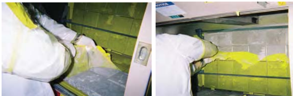
Figure 5-2. Stripcoat Removal
