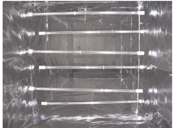
Figure 2-2. Device installed inside the test rig. There are 6 lamps. A reflective surface was placed in the duct.
