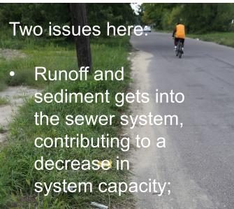
Eroded soil eventually clogged outlets, led to flooding in the roadway
