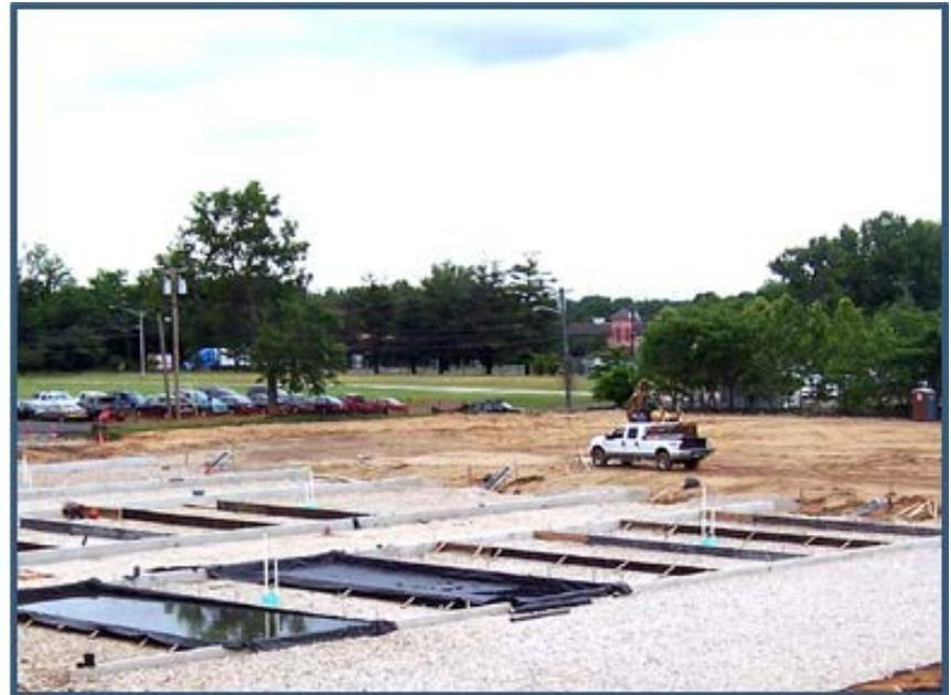
**Infiltrate drains from the lined sections to 1,500-gallon tanks on the east side of the parking lot where it can be sampled.**
