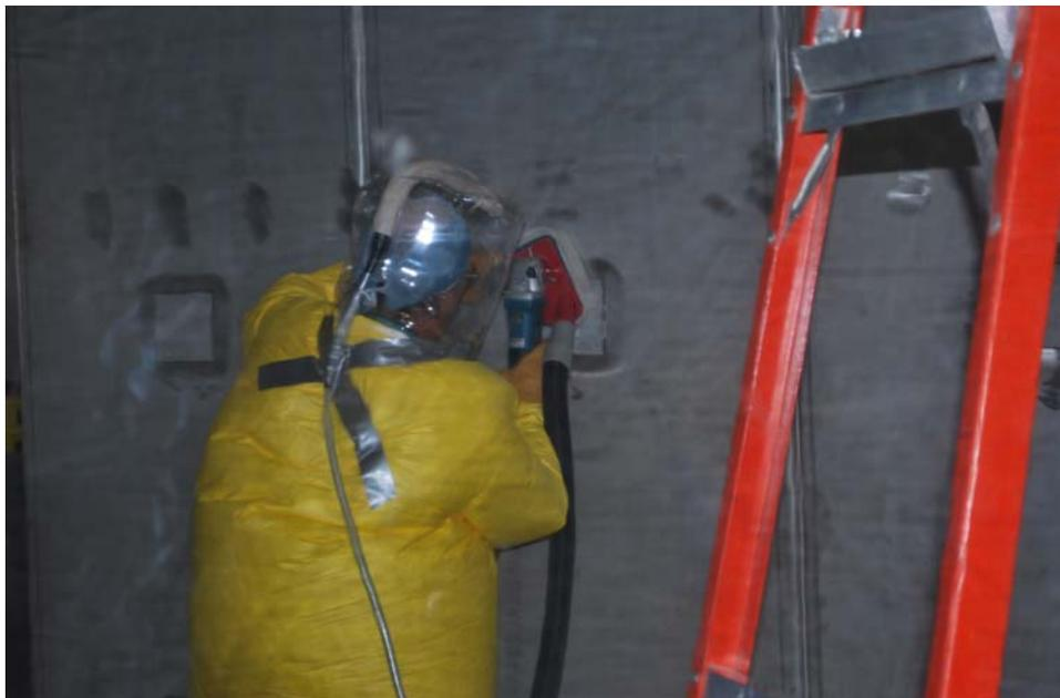
**Figure 3-3. SDG-DMD being applied to concrete coupon.**
