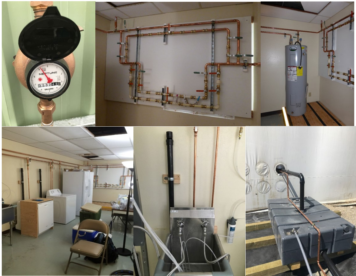
Figure 4: Premise plumbing setup at the WSTB: the water meter outside the building (top left), premise plumbing pipes (top middle), water heater (top right), dishwasher, washing machine and refrigerator (bottom left), utility sink (bottom middle) and exterior tank (bottom right).
