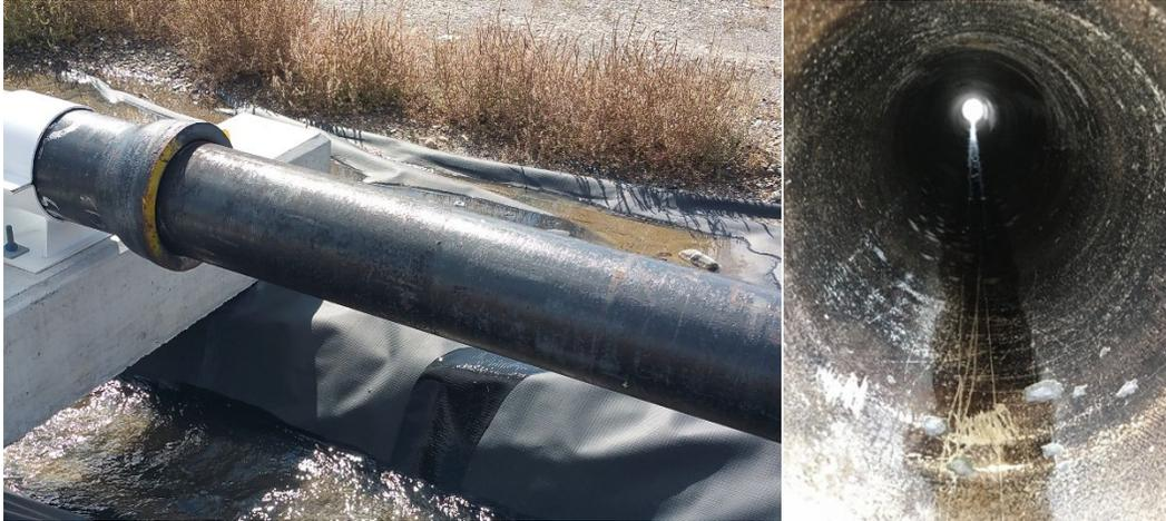
**Figure 6: External and internal view of the cement-mortar lined pipe.**
