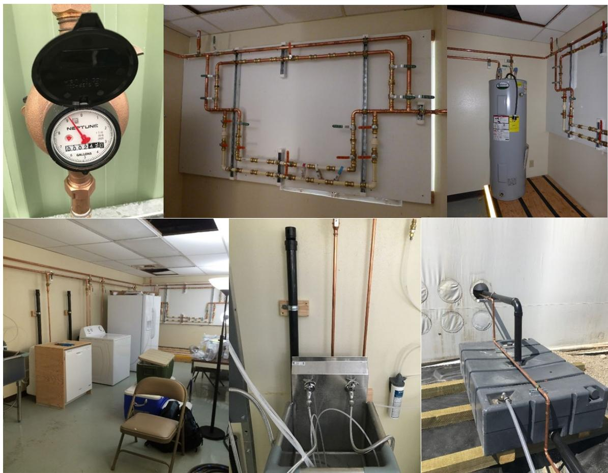
**Figure 5: Premise plumbing setup at the WSTB: the water meter outside the building (top left), premise plumbing pipes (top middle), water heater (top right), dishwasher, washing machine and refrigerator (bottom left), utility sink (bottom middle) and exterior tank (bottom right).**
