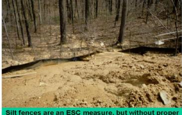
Silt fences are an ESC measure, but without proper installation and maintenance, they are worthless.
