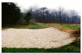
Infiltration trenches allow stormwater to percolate slowly into the soil.
