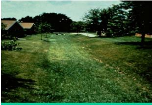
Grassed channels are effectively used along roadways to convey and infiltrate stormwater.
