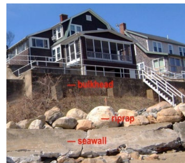
Figure 4-38. Example of a hardened shoreline.
