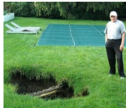
Figure 4-14. Photo of a collapsed cesspool after a recent rain event. Photo credit: Russell Beal; Source: Trauring (2013).
