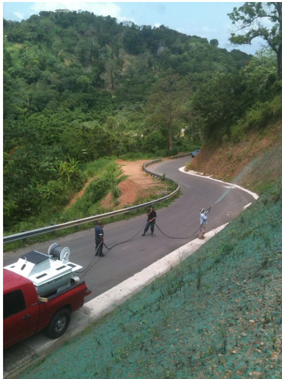
Figure 5-12. Protectores de Cuencas and Ridge to Reefs Inc., hydro-seeding a steep slope along the side of a mountain road in the Guánica Bay Watershed (photo provided by Paul Sturm)
