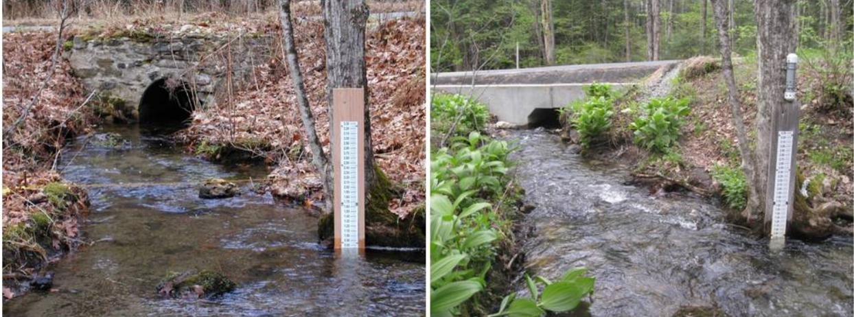
Figure 29. A culvert replacement downstream of a stream gage on Gulf Brook in Pepperell, MA caused enough of a channel change to necessitate a new rating curve.
