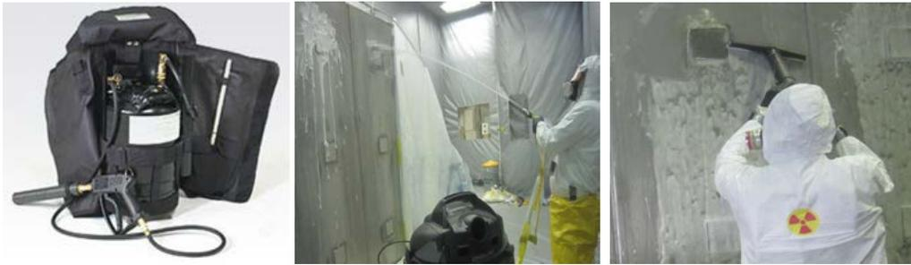
**Figure 3-3. Foamer, foam application, and vacuum removal.**
