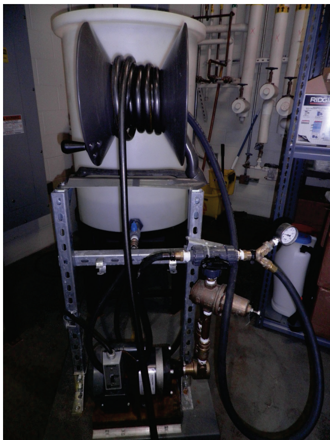
Figure D-7: DI water supply system
