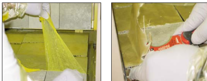
Figure 3. Removal of Stripcoat TLC Free TM (left) and Removal of Orion TM SC (right)
