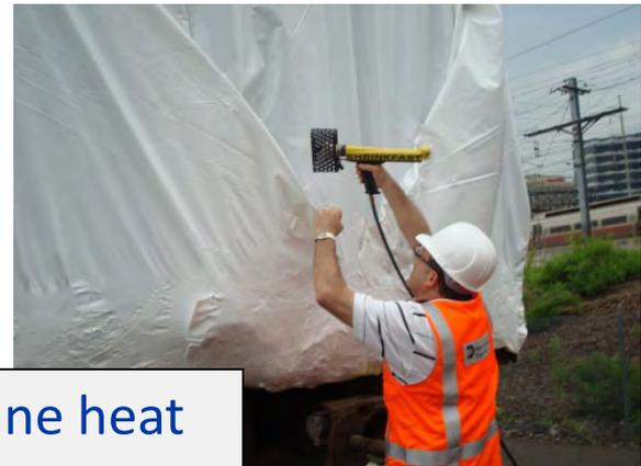
Using propane heat gun to seal seams
