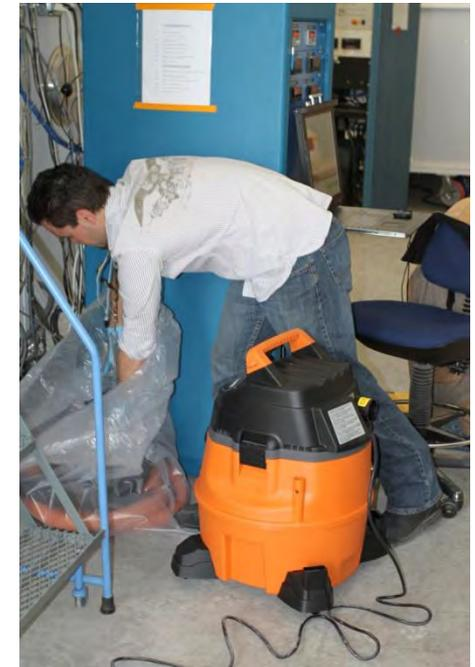
Pre-cleaned all surfaces using a HEPA-filtered vacuum.
