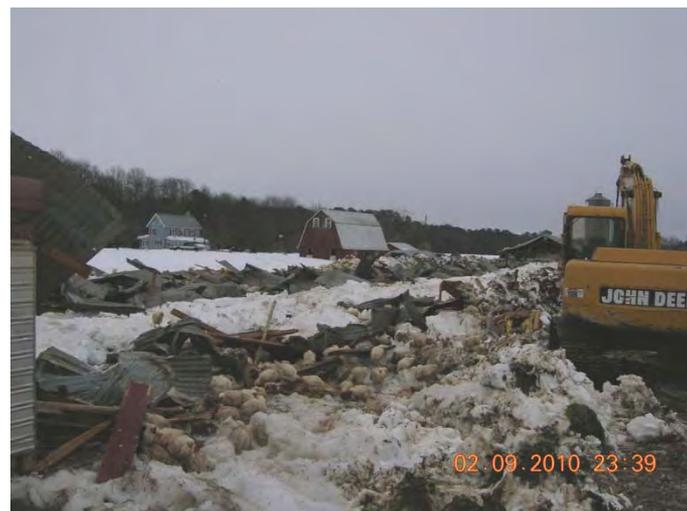
Excavator removing part of the roof to allow access.
