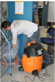
Pre-cleaned all surfaces using a HEPA-filtered vacuum. Filters were disposed of as hazardous waste.
