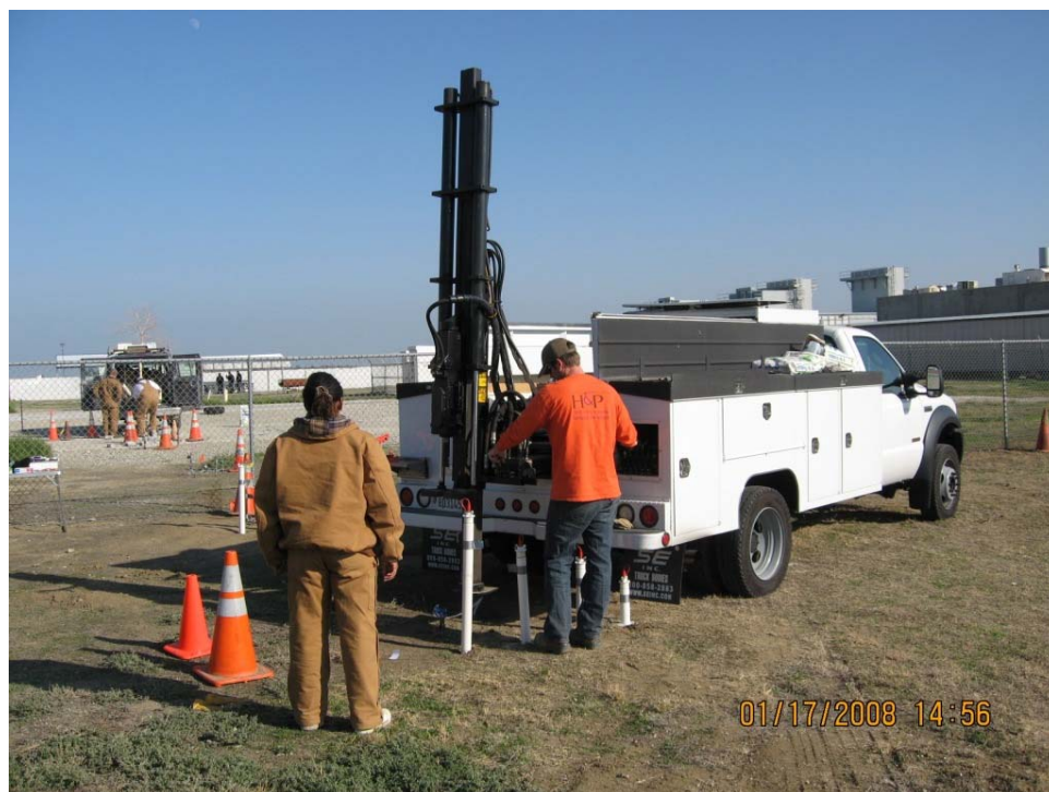
Photograph 4: Installation of PDS wells.
