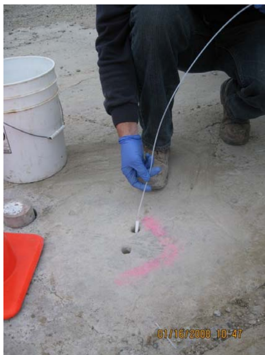
Photograph 6: Installation of sub-slab soil gas probe.
