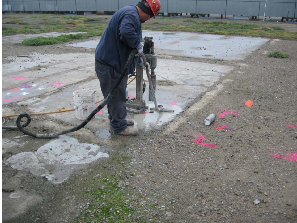
Photograph 1: Concrete coring at Building 173 slab.
