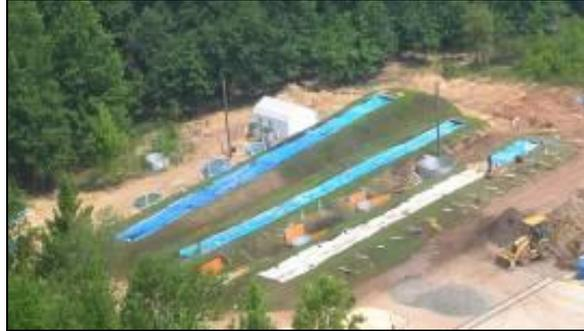
**Figure 1.** Construction of the 5%, 1%, 0.5% swales (from left to right).
