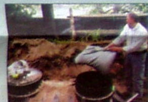
One alternative to an OBD is a recirculating biological filtration system.
