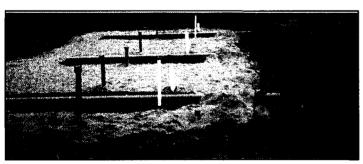
An SAS during construction. Each trench receives a fourth of the discharge from each test replicate. Dosage is 0.74 gallons per sq. ft. per day.
