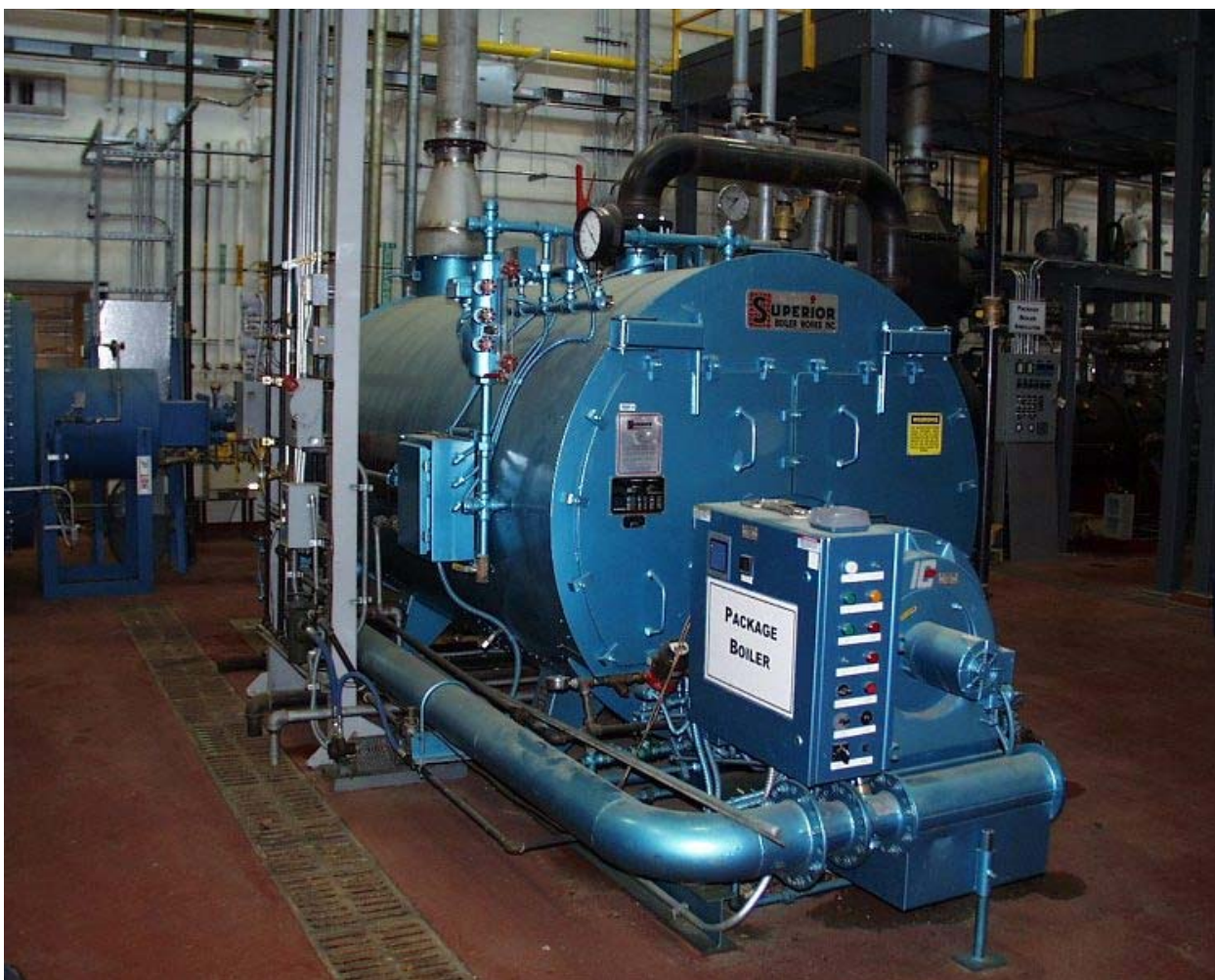
Figure 2. Photograph of the burner end of the firetube package boiler used in the biofuel tests.
