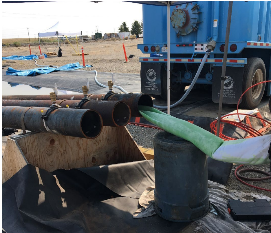
Figure 16: Resin soaked CIPP sock being pulled through the iron pipe.
