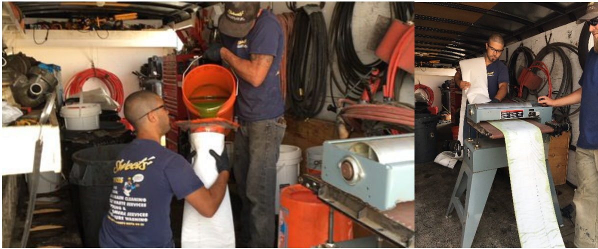
Figure 15: Flexible CIPP fabric sock being soaked in resin.
