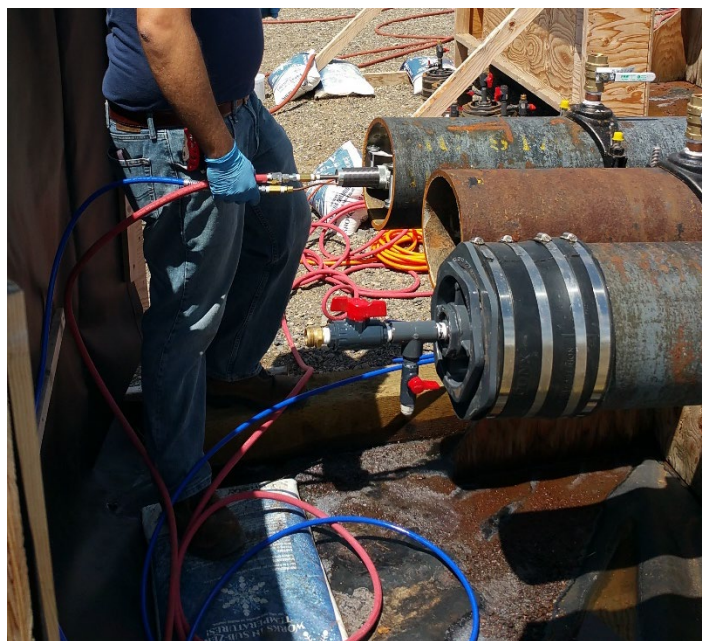
Figure 12: Rotary air sprayer inserted into the pipe to apply the DragX coating.
