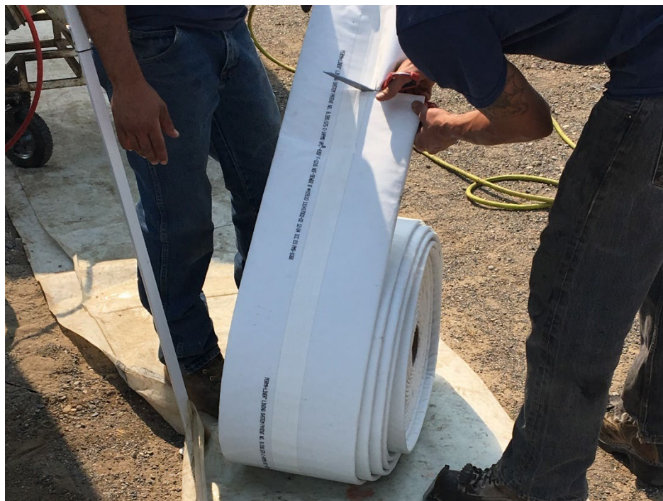
Figure 14: Flexible CIPP sock being cut to the length of the iron pipe.
