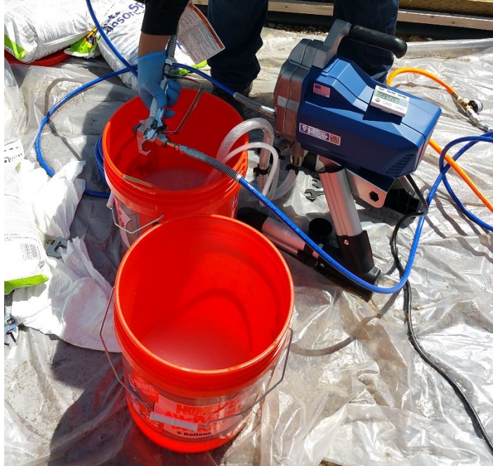
Figure 11: Mixing the Oceanit DragX coating in a bucket.
