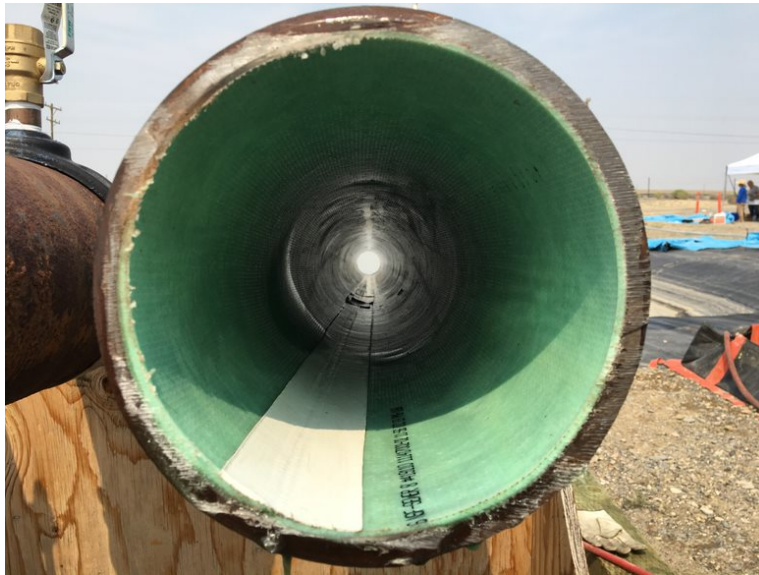
Figure 18: Finished CIPP sawed off to the length of the iron pipe.
