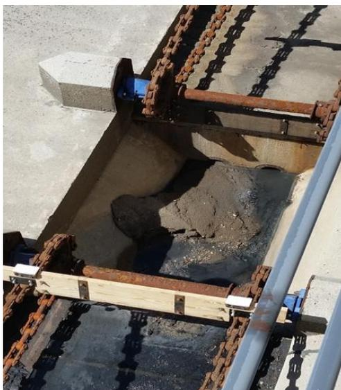
**Figure 4. Close-up view of the collection trench in a drained aeration grit tanks showing potential for Cs contaminated sediment accumulation and concentration.**
