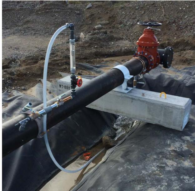
**Figure 3. Water Security Test Bed system flow regulator.**
