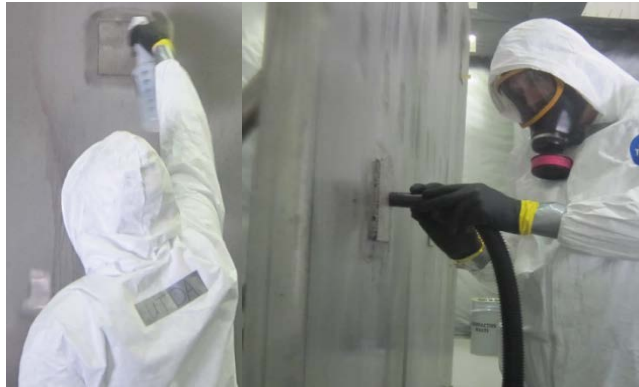
Figure 5-1. Application and removal of ND-75 or ND-600.
