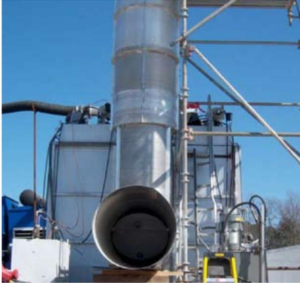
**Figure 2-8.** Stack Dilution Inlet
