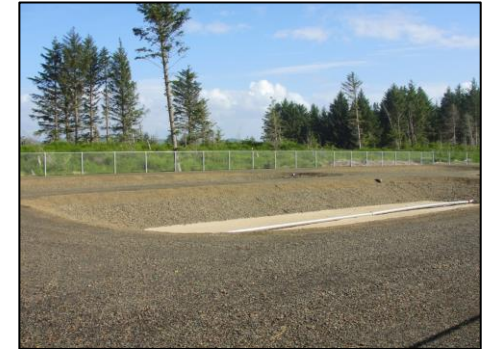
WWTP Rapid Infiltration
