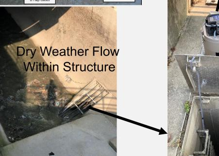
Remote Composite Sampler ~10L between 8-11 am ~500 ml every 15 min
